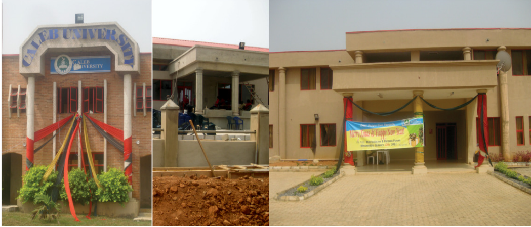
Doric Columns Featured on Caleb Site
